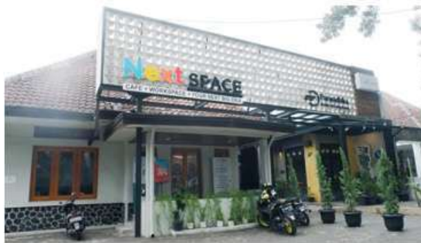
Fig. 10. Nextspace (Front View)
